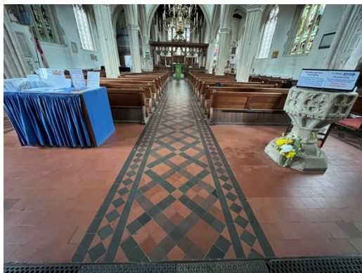
Image 3.11: Victorian tiled floor to the nave
