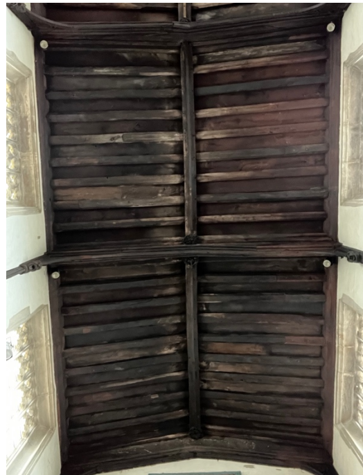
Image 3.5: Roof above the nave
