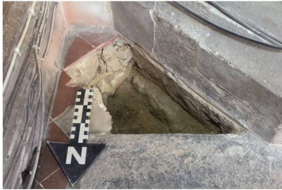
Fig. 5 Views of Test pit 2 (left) and Test pit 5 (right, showing ledger and limecrete screed, with pier foundation, scale 0.15m
