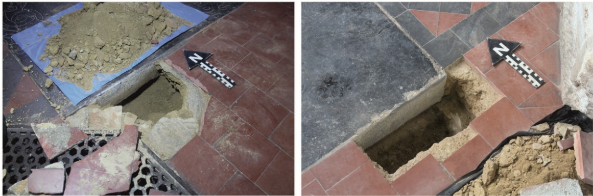
Fig.3 Views of Test pit 1 (left) and Test pit 6 (right, showing ledger and limecrete screed, with pier foundation, scale 0.15m
