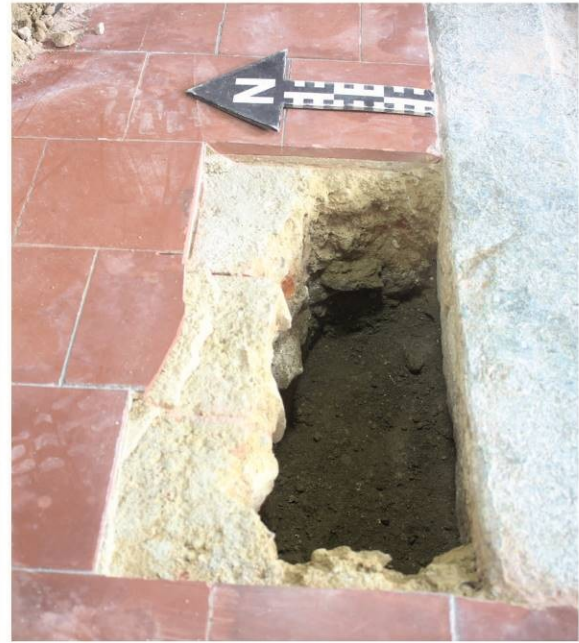
Fig. 5 Views of Test pit 2 (left) and Test pit 5 (right, showing ledger and limecrete screed, with pier foundation, scale 0.15m
