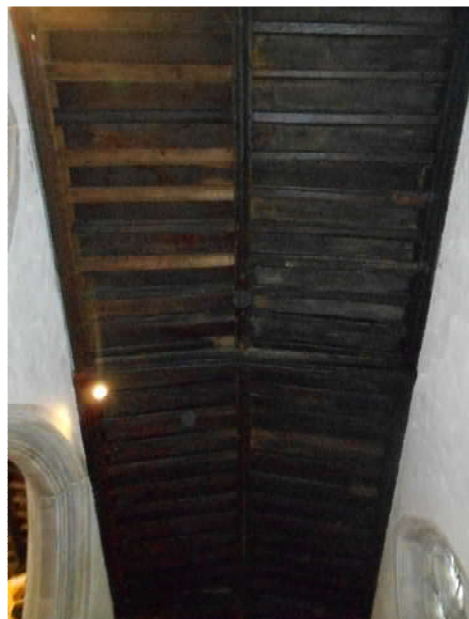
North aisle ceiling
