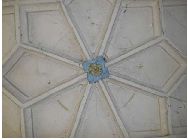
Ribbed vaulting to north porch ceiling
