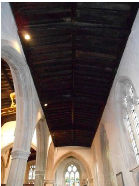
South aisle ceiling
