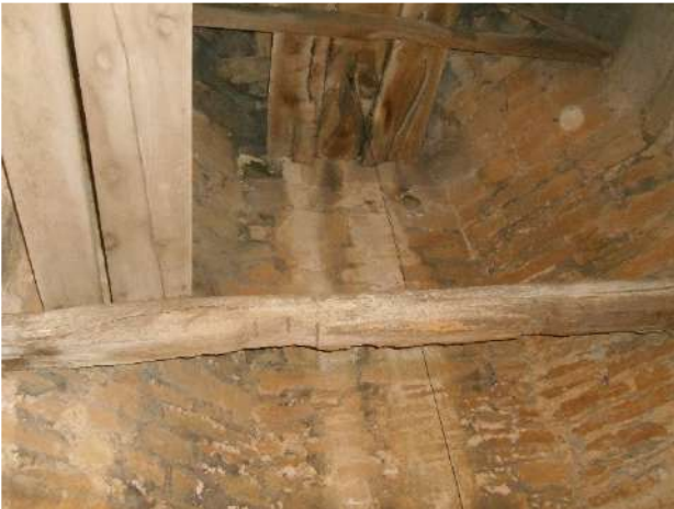
View looking up inside the spire with cross members and partial boarding in two stages
