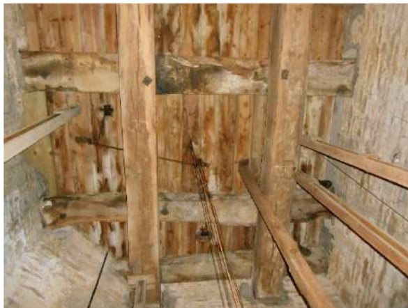
View looking up inside the spire with cross members and partial boarding in two stages
