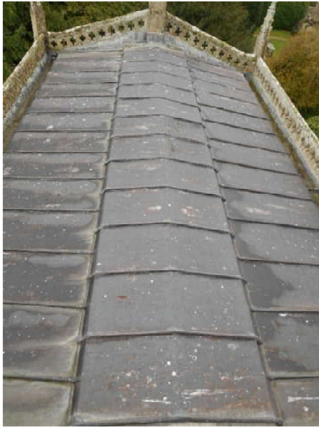
View across chance roof, with stepped ridge, looking east from nave roof. Debris build-up to both parapet gutters
