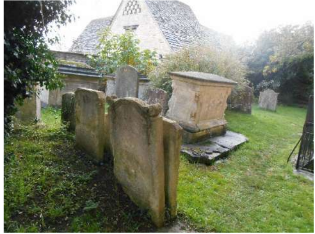
Example of uneven ground levels impacting upon condition of some chest tombs in churchyard (photo south side of church, by boiler room railings)
