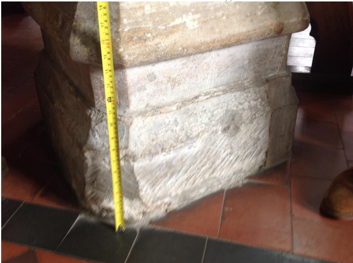
Photograph C2: Base of internal columns showing undressed stone indicating a higher floor level pre 1882 suggesting the original stone floor was at a higher level before the 1882 re-ordering.
