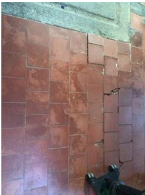
Many of the tiles are damaged by point loading (see below) or by a lack of adhesion to the limecrete floor.
