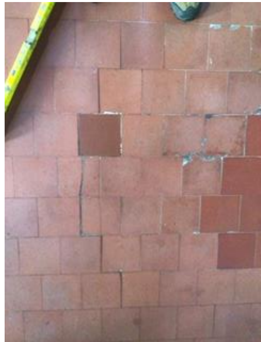
Many of the tiles are damaged by point loading (see below) or by a lack of adhesion to the limecrete floor.
