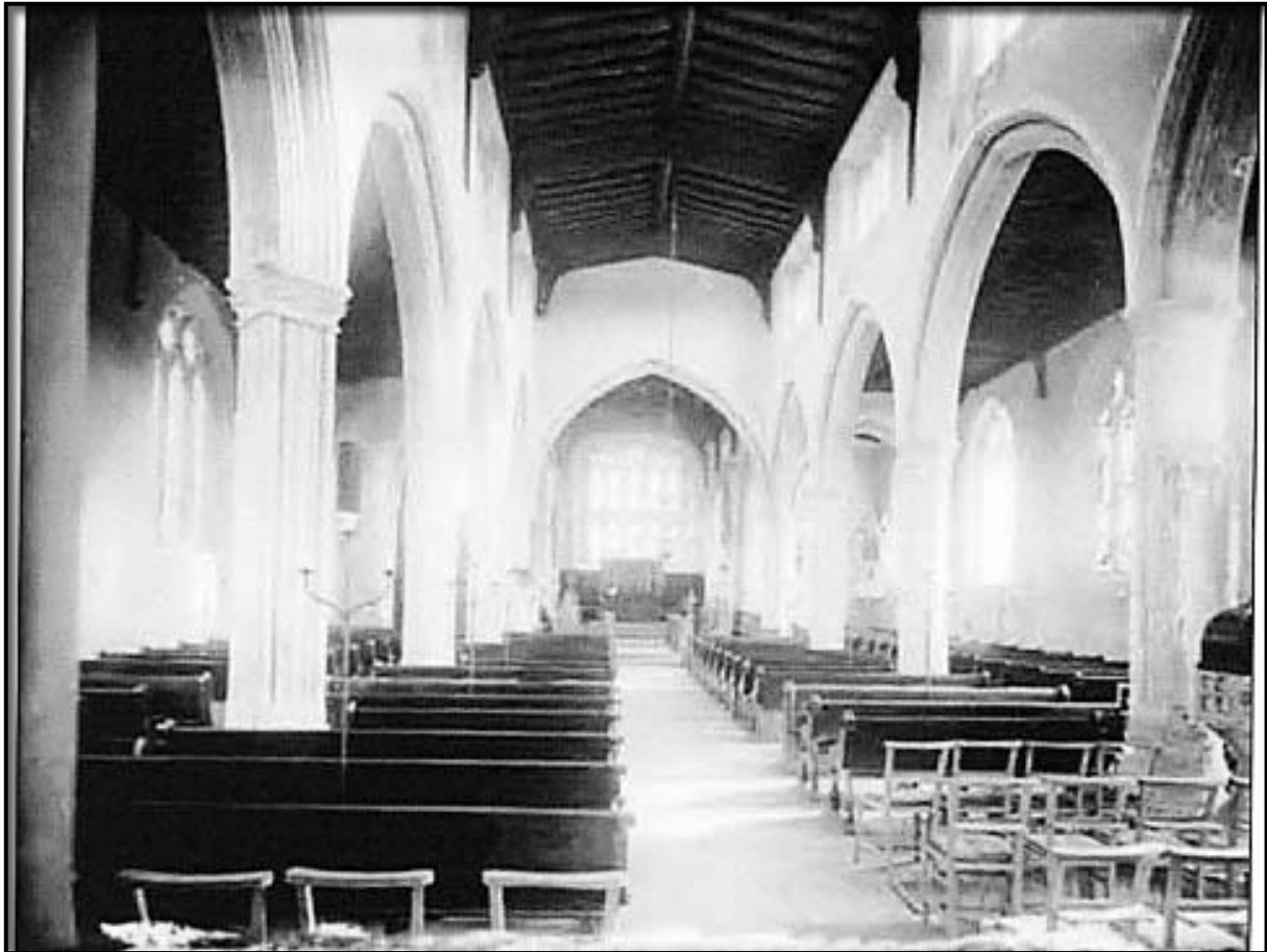
View looking east from the chancel, circa 1882; this was post reordering and before the screen was installed. Note the clear and unobscured view to the altar and east window
