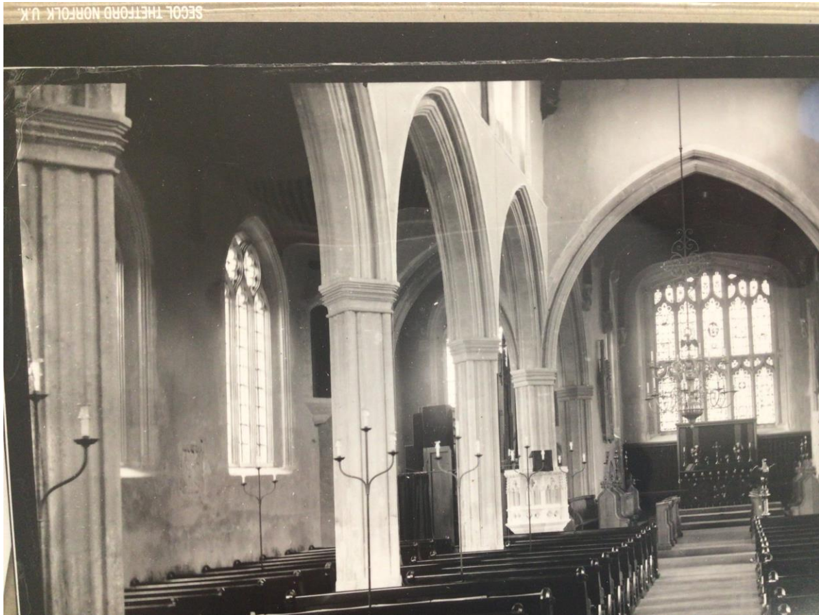
View from the west end into the chancel post 1882 reordering but before the screen was installed (note the George IV Coat of Arms is not in position above the chancel arch)
