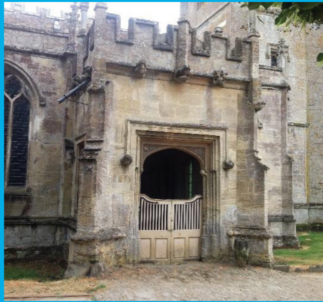
▲ existing closed north porch.
