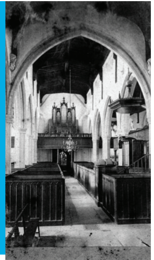
▲ The 1828 reordering looking west - note the organ on the balcony, box pews and stone floor (higher than it is today).
